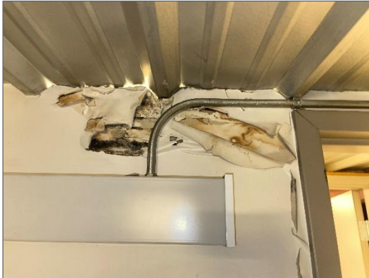
Photo 12 - Mould-impacted and water damaged drywall wall finishes along south wall.
