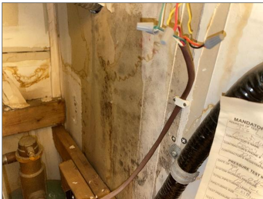
Photo 9 - Mould growth on north drywall wall.
