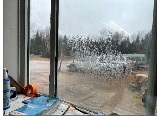
Photo 4 - Condensation on exterior glass windowpanes.
