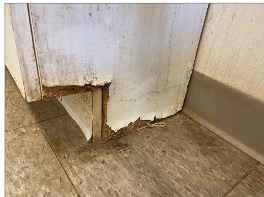
Photo 8 - Water damaged wood cabinet.
