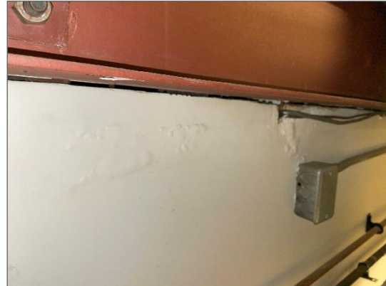
Photo 13 - Bubbling paint along west drywall wall.
