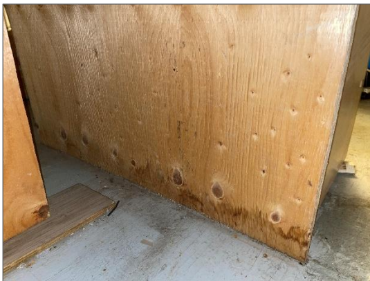
Photo 14 - Water stained wood shelving.
