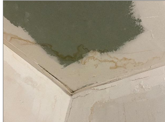
Photo 6 - Water stained and water damaged drywall ceiling.
