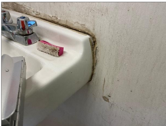
Photo 7 - Water damaged drywall present behind the sink.
