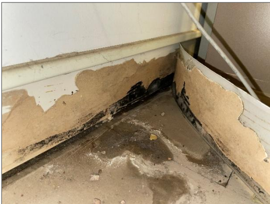
Photo 1 - Mould growth on drywall wall finishes along the west wall. Efflorescence and water stains also present on the vinyl floor tiles below.
