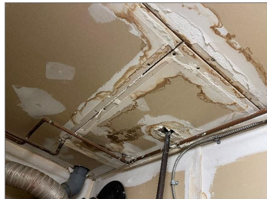
Photo 10 - Water damaged and water stained drywall ceiling.
