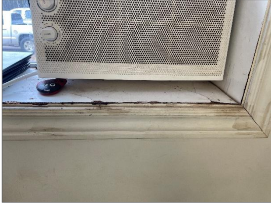
Photo 3 - Water damaged and swollen wood windowsill.
